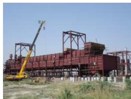
Diffuser under construction
